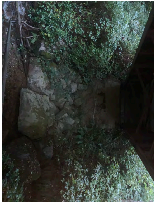
Right Bank Abutment when facing downstream
